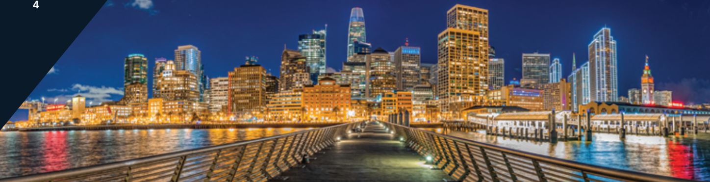
Salesforce Tower (center) and Embarcadero Center (right), San Francisco, CA
